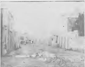
Wilhelmina Street has also had its face lifted. The old picture above shows that 25 years ago muddy roads and lack of sidewalks presented a problem. Although the fine and durable home on the right side of the street remains the same, many new buildings have been added. The picture
